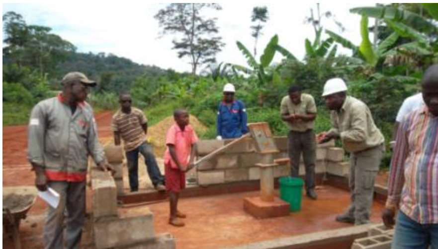
Figure 7: Installation of Community Water Bores at Mbalam Village
