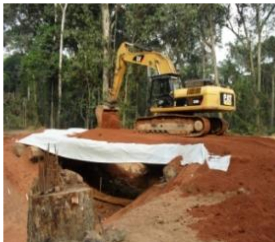
Figure 9: Construction of a Bridge on the Road to Nabeba
