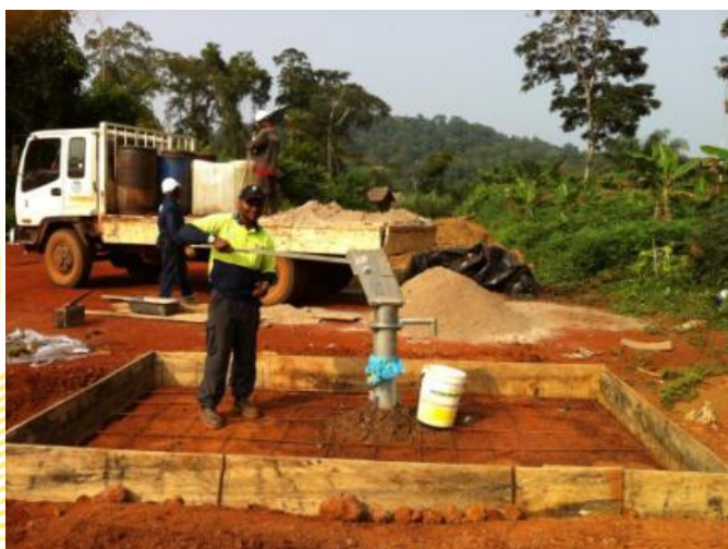
FIGURE 4: INSTALLATION OF COMMUNITY WATER BORES AT MBALAM VILLAGE
